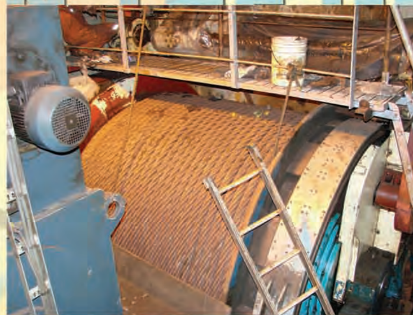
Saipem驳船上平顺的绳槽。 Smooth spooling for Saipem's barge.
